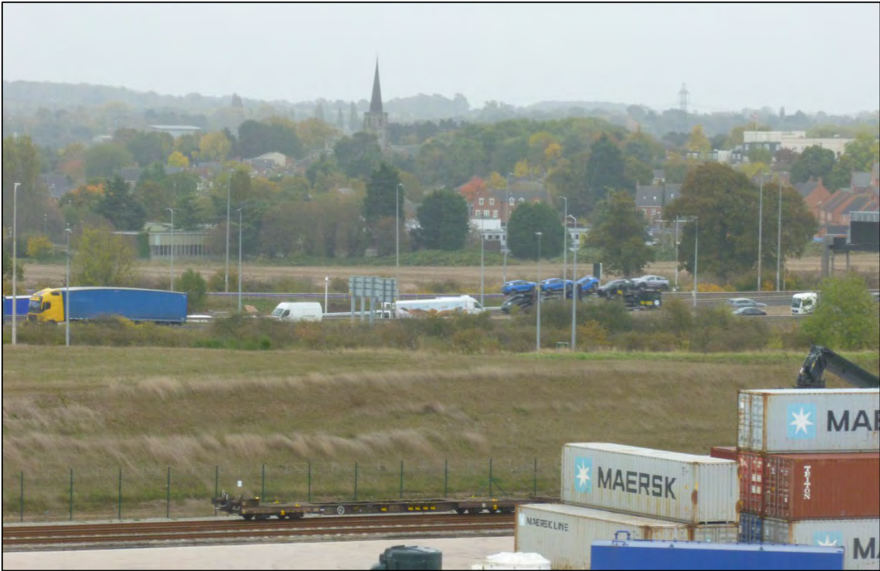
Plate 11 - View of tower and spire of Church of St Andrew, Kegworth from bund to northwest of EMG1 Works.
